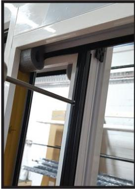
Re-fit the plastic interlock screws – these pick up on the back of the cover trim and secure it in place
