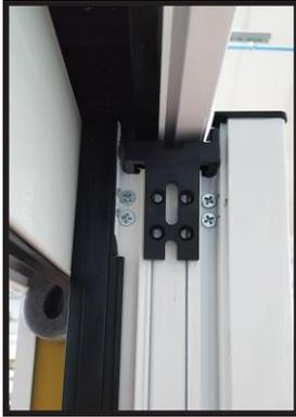
Fit the first door onto the track – DO NOT glaze at this point
